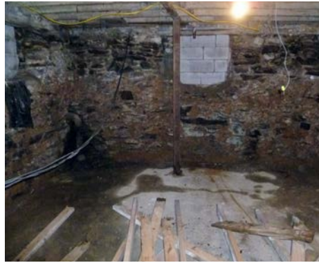
(Left) Pre-retrofit wet basement. (Right) Post-retrofit dry basement through the use of ccSPF against the stone foundation and a stand-alone dehumidifier. Ideally a sub-slab capillary break would be incorporated as well.
