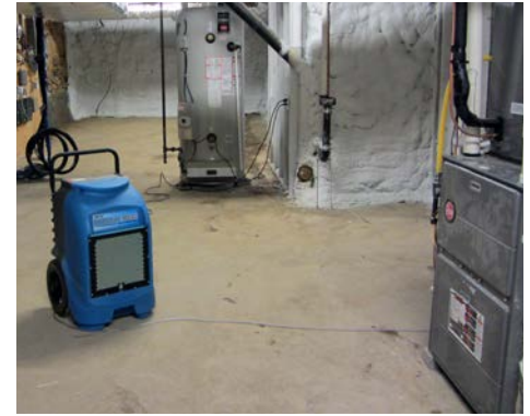
(Left) Pre-retrofit wet basement. (Right) Post-retrofit dry basement through the use of ccSPF against the stone foundation and a stand-alone dehumidifier. Ideally a sub-slab capillary break would be incorporated as well.
