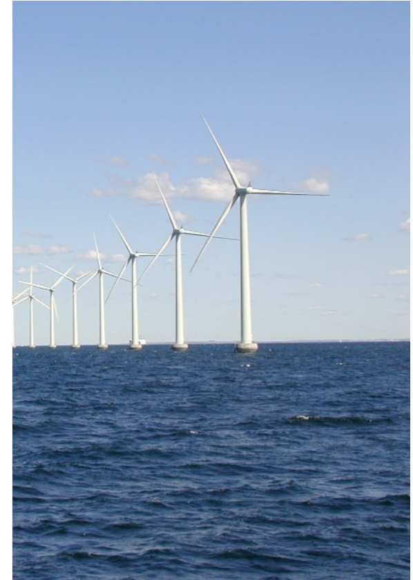
Photo from HC Sorensen, NREL 17856
