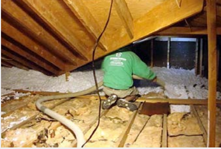
Contractors install blown insulation in the attic.
