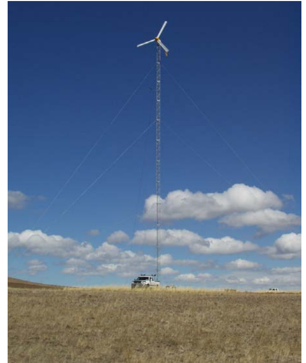
Bergey Excel 10, 10-kW turbine, Klickitat County, Washington Photo by Gwen Bassetti, NREL 26429
