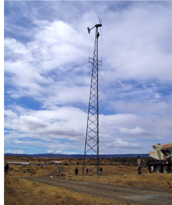
Bergey Excel 10, 10-kW turbine; Ellensburg, Washington Photo by Randy Brooks, NREL 29553
