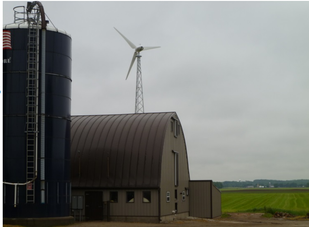
Endurance E3120 turbine; 50-kW turbine, Appleton, Wisconsin Photo by Kettle View Renewable Energy, LLC, NREL 28428
