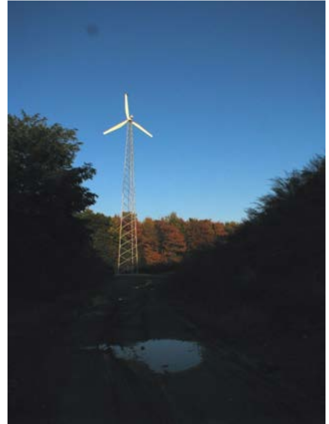
Entegrity EW50, 50-kW turbine, Kittery, Maine
