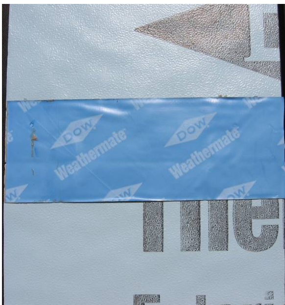
Figure 42. Dow Weathermate butyl on ffPIC— large test
