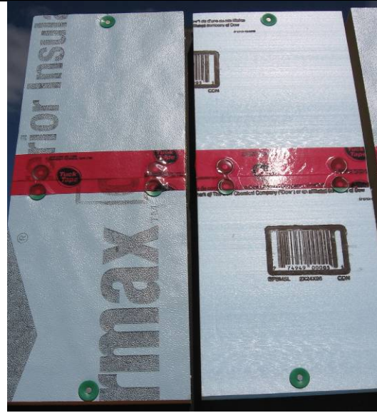
Figure 28. Tuck tape on ffPIC (left) and XPS (right)
