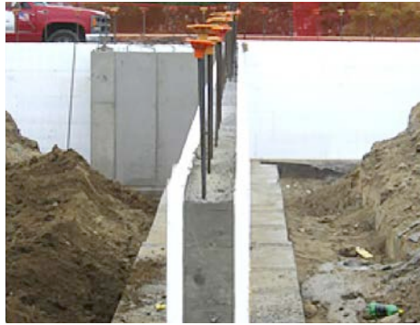
ICF wall construction
