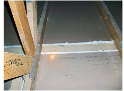
Air-sealed top plates before attic insulation
