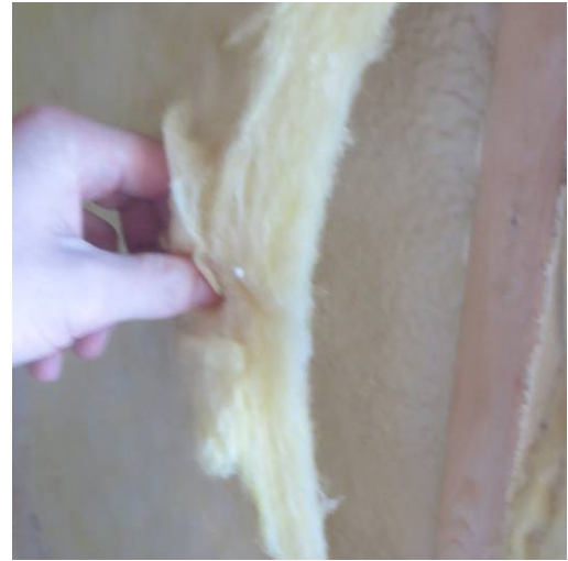
Figure 4. Flash and batt of 2 × 4 wall cavity
