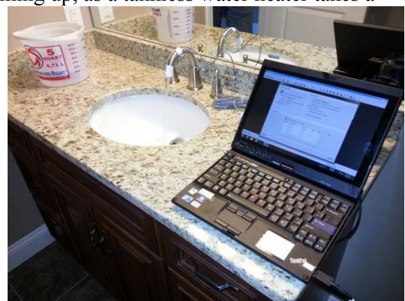
Figure 20. DHW monitoring setup
