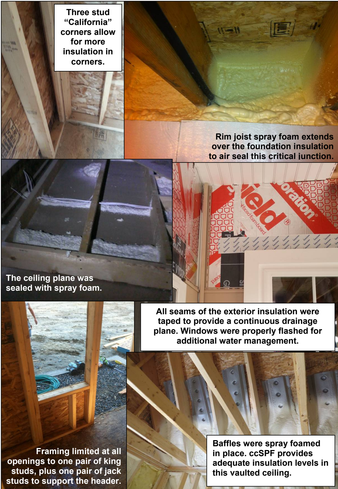
Figure 16. Several critical building envelope details
