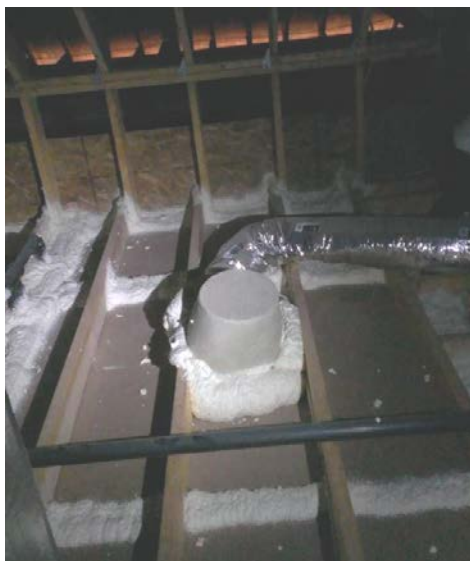
Figure 8. Critical air seal of ceiling plane
