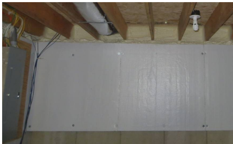
Figure 6. Air sealing critical transition between sill plate and foundation wall
