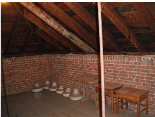
Figure 5. Top floor of building before renovation
