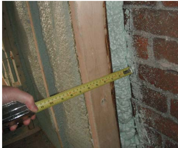
Figure 4. Partially insulated wall
