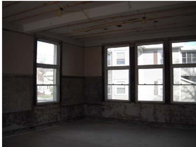
Figure 7. Old windows were replaced with new triple-pane windows
