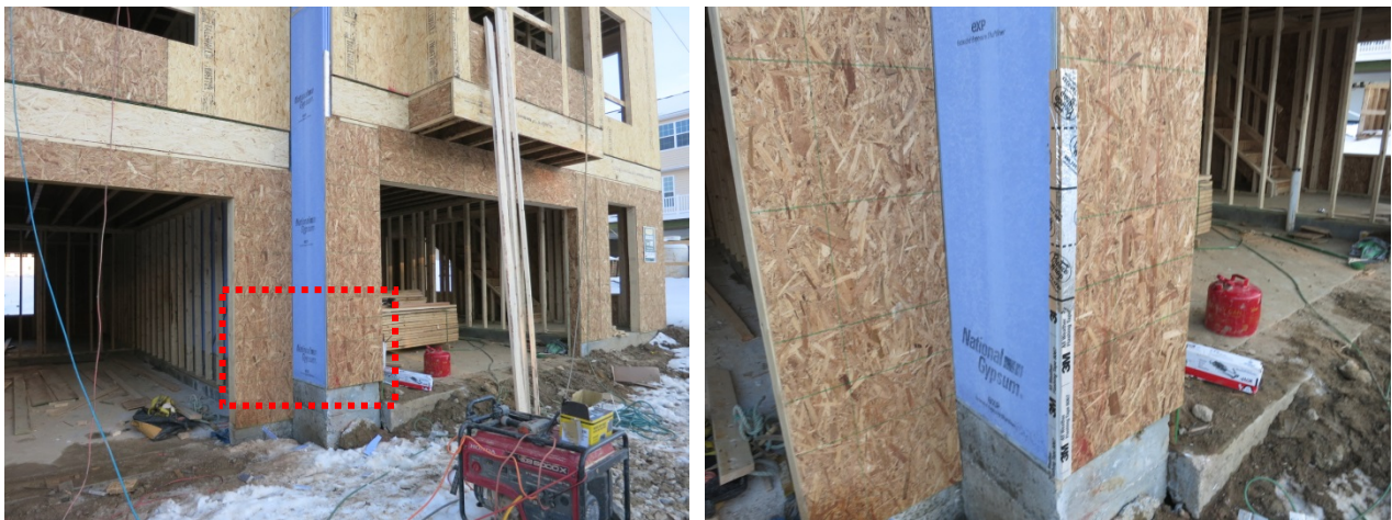
Figure 75. Test application of two types of adhesive sheathing tape
