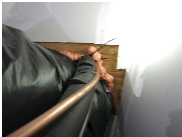
Figure 72. Ceiling and wall penetrations at mechanical room (Unit 6702)
