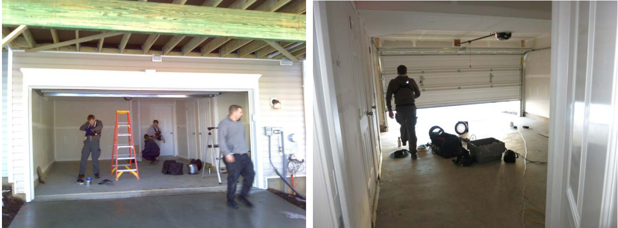
Figure 67. Unit 6706 garage overview
