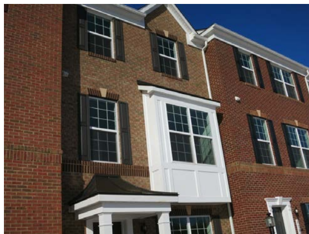
Figure 30. Front bump out bay detail at unit 6702
