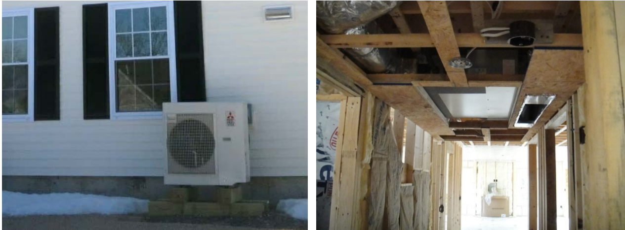
Figure 78. MSHP 3:1 outdoor unit (L) and indoor ceiling recessed air handler (R)
