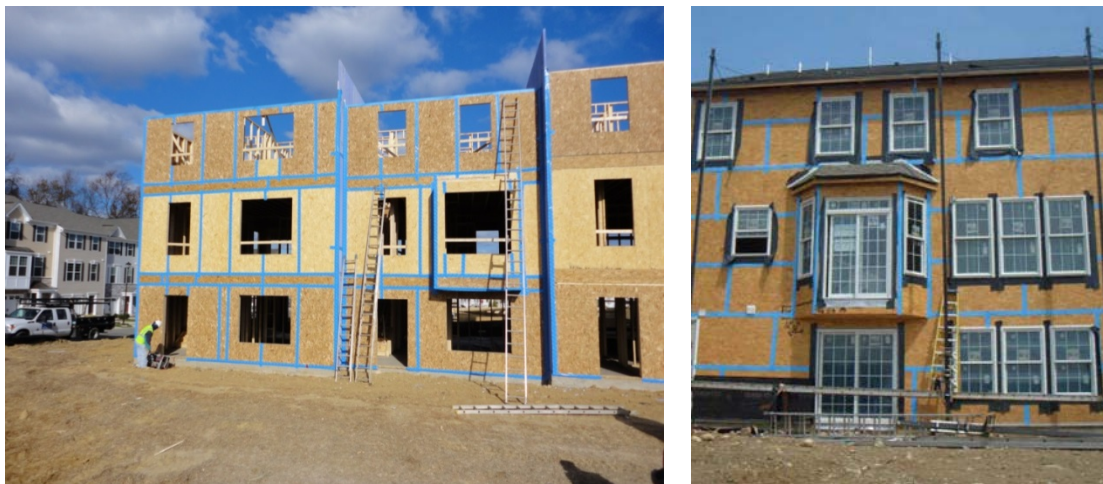
Figure 17. Taped seams of exterior sheathing and gypsum fire separation wall
