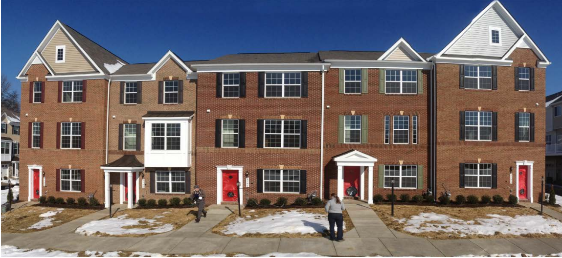
Figure 19. Setup for multifan air leakage testing (Day 2)
