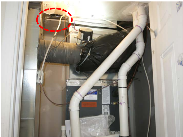
Figure 73. Ceiling penetrations at mechanical room (Unit 6702)
