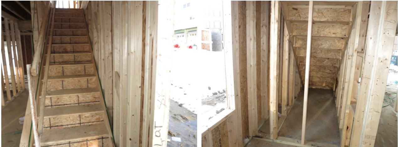
Figure 77. Stairwell on exterior wall
