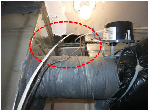
Figure 73. Ceiling penetrations at mechanical room (Unit 6702)
