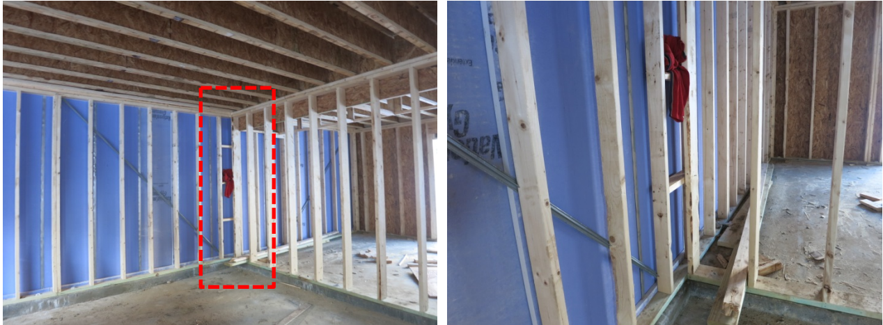
Figure 52. Garage tee wall intersection, showing ladder blocking
