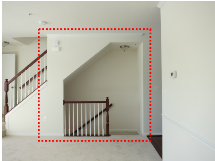
Figure 50. Air leakage at stair landing (first-to-second floor)
