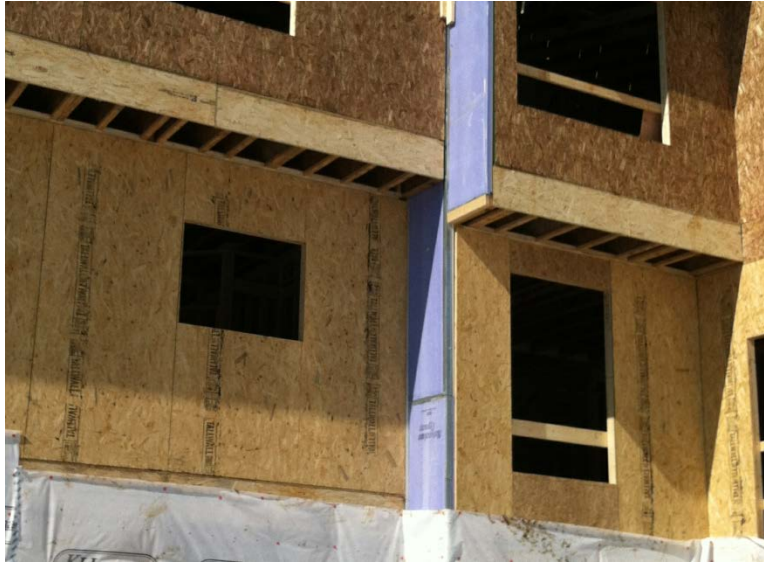
Figure 60. Separation wall “jog” at second and third floors, frame building
