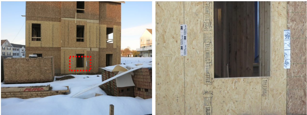
Figure 74. Test application of two types of adhesive sheathing tape
