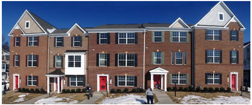
Front elevation, set up for multifan "guarded" testing.
