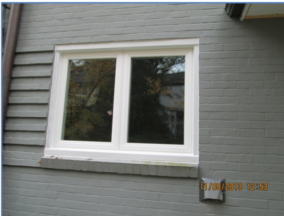
Figure 27. Replacement window in FB unit
