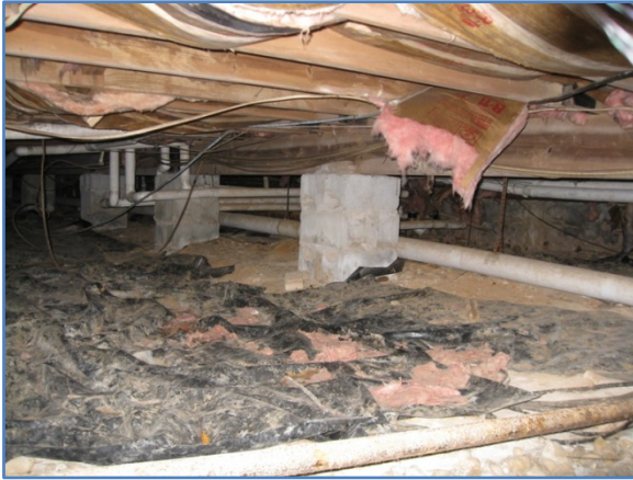
Figure 7. FV building crawlspace prior to upgrades
