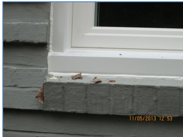
Figure 28. FB replacement window—flashing and caulking
