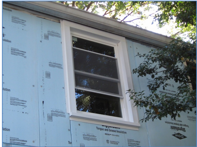
Figure 33. Replacement window installed and flashed
