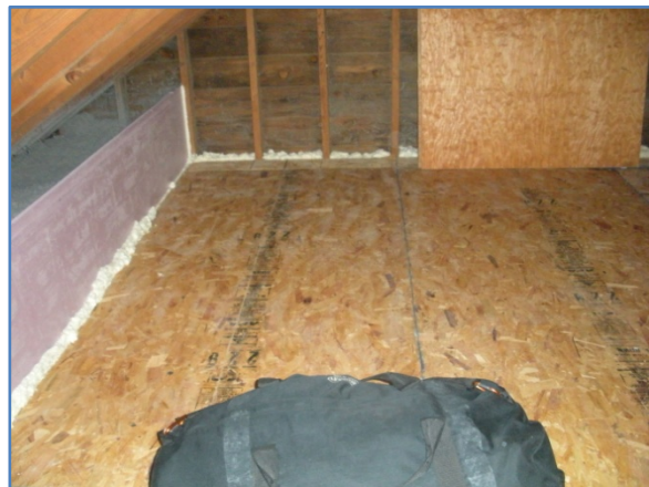
Figure 17. Completed attic retrofit
