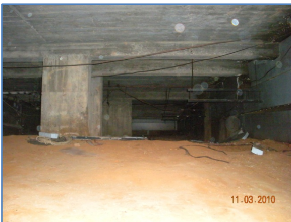
Figure 9. B building crawlspace prior to upgrades
