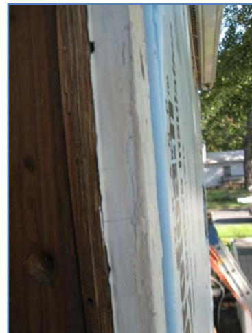
Figure 31. Foam board extends beyond original window trim
