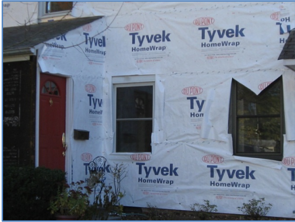
Figure 36. WRB installed over foam sheathing (not shown)
