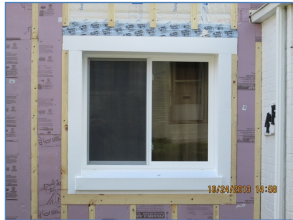
Figure 21. Window flashing integrated with foam insulation
