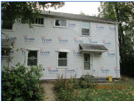
Figure 41. WRB installed over foam sheathing
