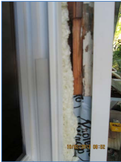
Figure 32. Additional window trim and foam sealing
