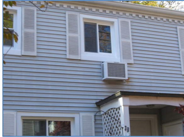
Figure 23. BV building with new windows and trim
