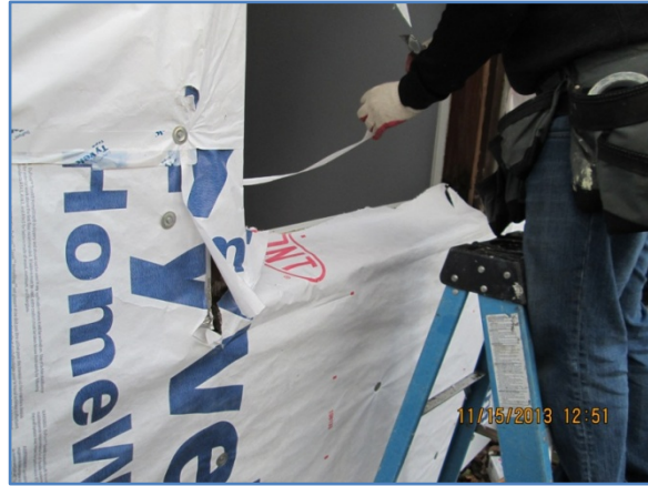
Figure 37. WRB wrapped into window opening
