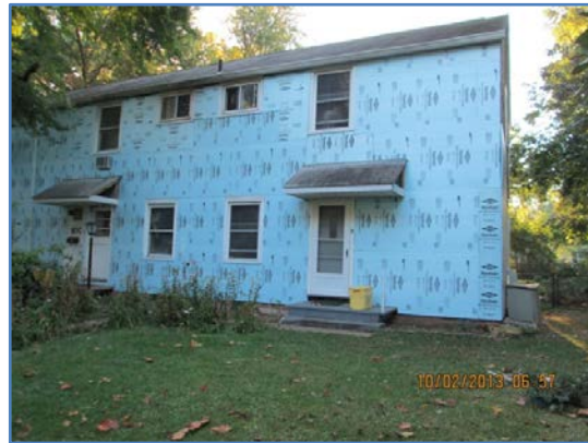
Figure 40. Foam sheathing installed
