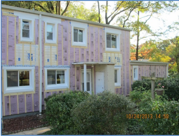
Figure 25. Block building with exterior insulation installed
