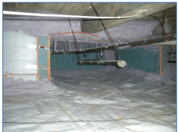
Figure 10. Building crawlspace after repair/retrofits
