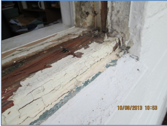
Figure 18. Window rough opening prior to window installation
