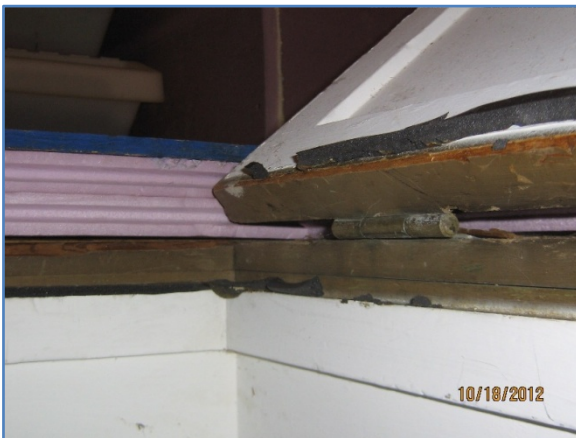
Figure 12. Foam board at attic storage area
