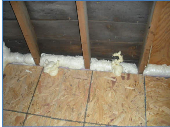
Figure 15. Gable end wall air sealing
