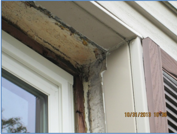
Figure 22. Replacement window installed in a BV unit
