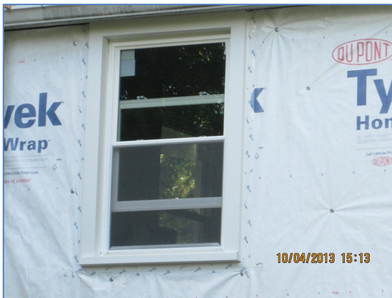
Figure 34. Additional window trim and foam sealing
