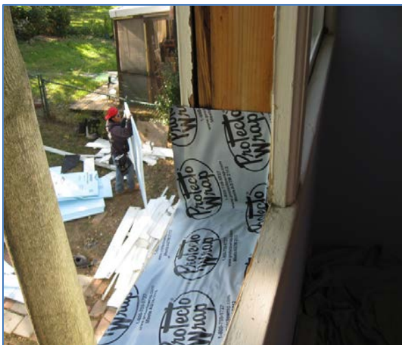
Figure 30. Window sill flashing on an FV unit
