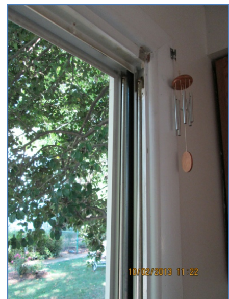
Figure 35. Replacement window installed and flashed
