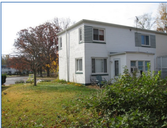
Figure 3. B building (1st home of 4 in set)
