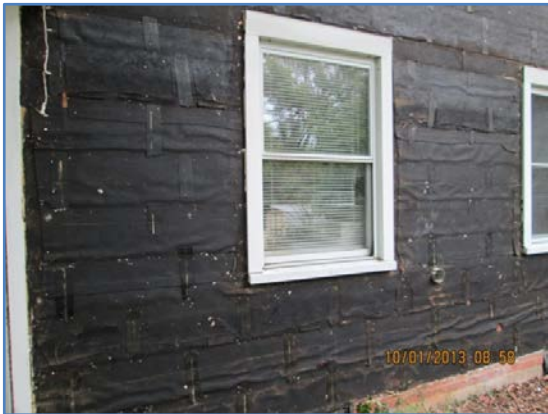
Figure 39. Original building paper on frame building
