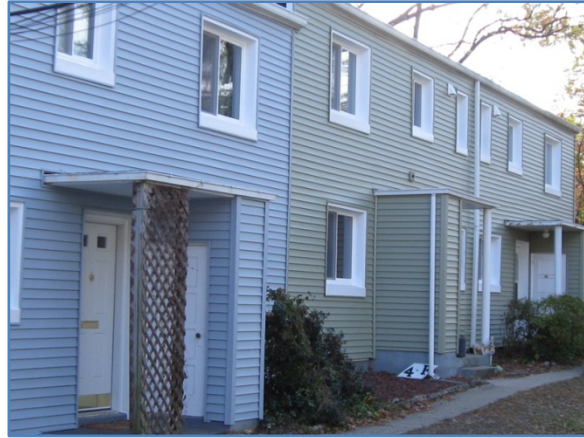
Figure 26. Completed block building with all energy upgrades installed
