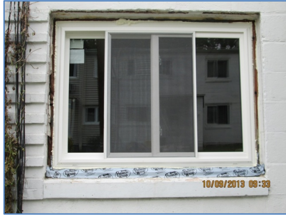
Figure 19. New replacement window installed over sill flashing and foamed
