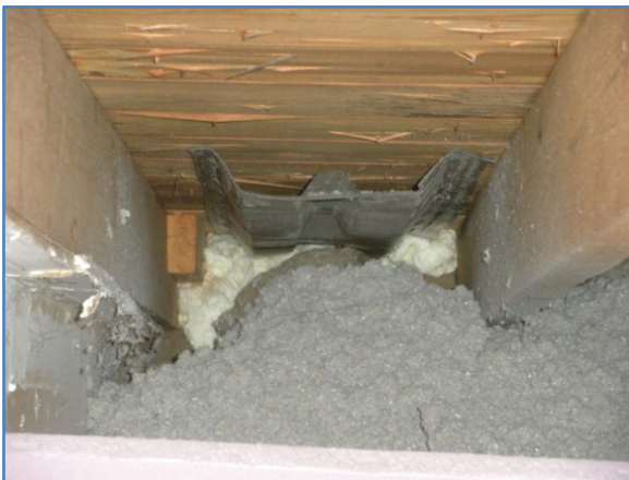
Figure 16. Exterior top plate air sealing
