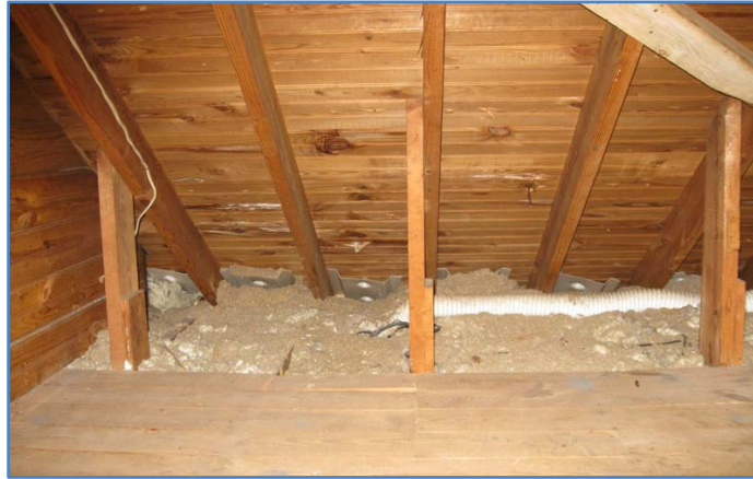
Figure 11. Typical attic of the wood-framed buildings
