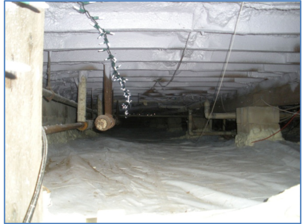
Figure 8. FV crawlspace after upgrades
