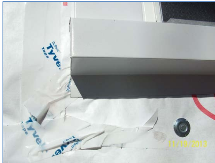
Figure 38. Window trim flashing integrated with WRB
