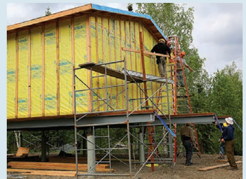
Galena, Alaska, where Yukon River flooding destroyed 90% of the buildings in 2013. Photo from Cold Climate Housing Research, NREL 32755
