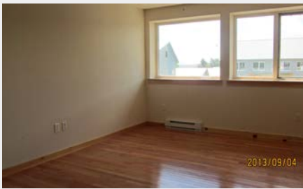
Loads were so small in these homes they only required 9 linear ft of electric resistance baseboard.
