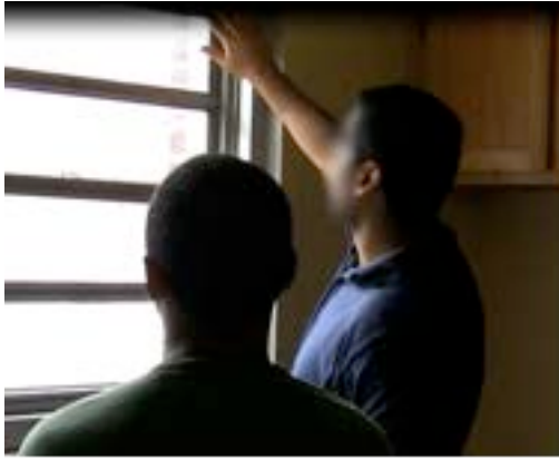
Figure 1. Testing of air leakage at window of public housing unit
