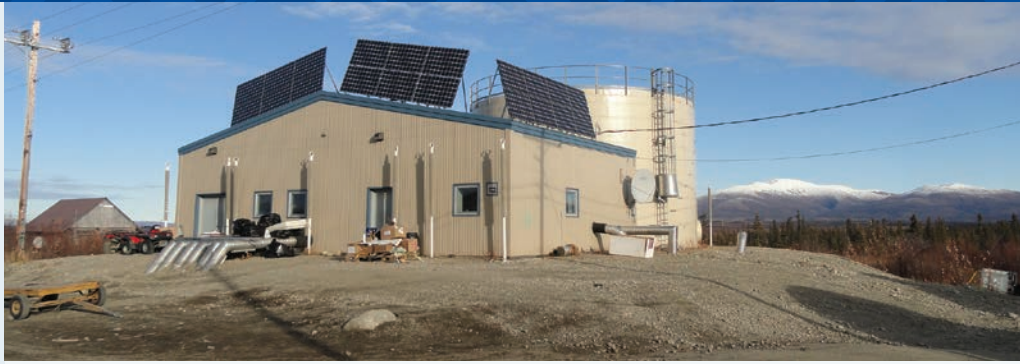
The Shungnak power plant is one of nearly 30 rural utilities the RUS team is visiting in 2015. Photo from Alaska Center for Energy and Power, NREL 33697.
