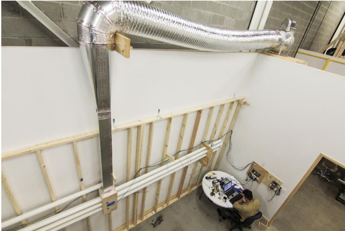
Figure 5. Testing a side outlet manifold configuration
