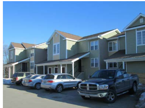
Figure 16. Building front after retrofit
