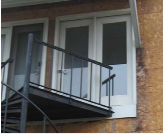
Figure 9. Rear patio doors and stairs at siding removal phase
