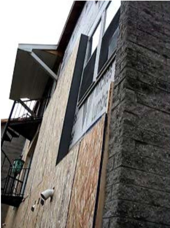
Figure 13. Rear windows prior to removal
