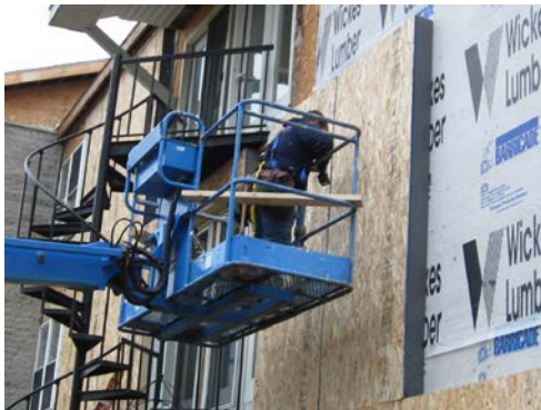
Figure 15. Installing a 6-in. retrofit panel
