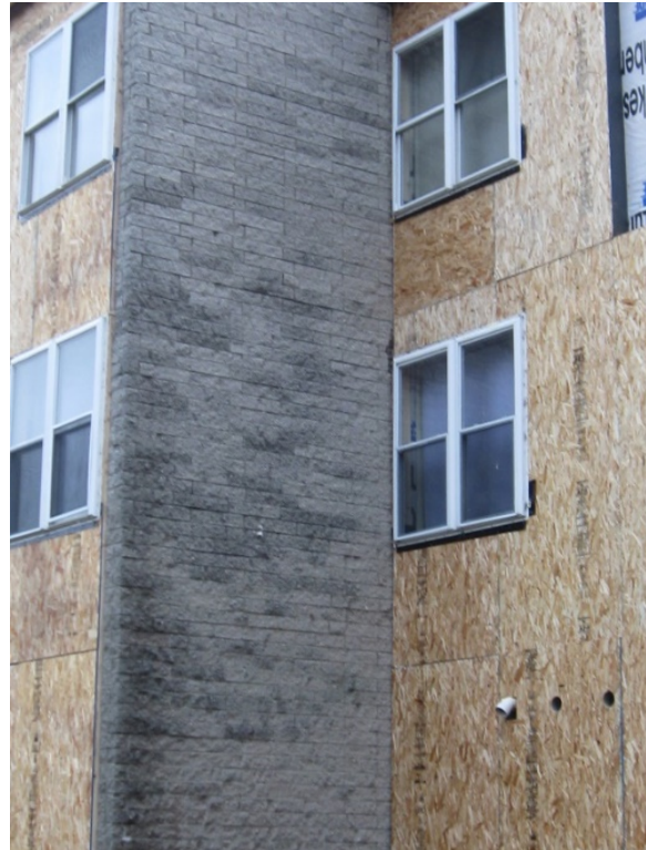
Figure 14. Rear windows after reinstallation
