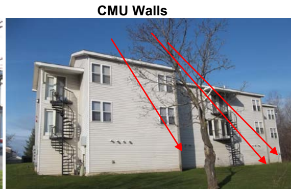
Figure 8. Building rear elevation, northeast
