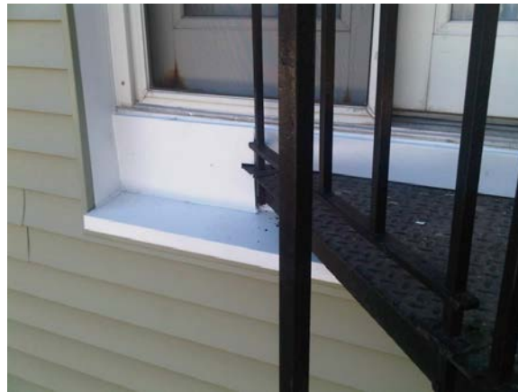
Figure 11. Completed rear entry at stair landing
