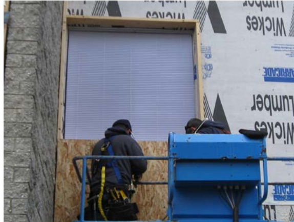
Figure 12. Framing installed around window opening
