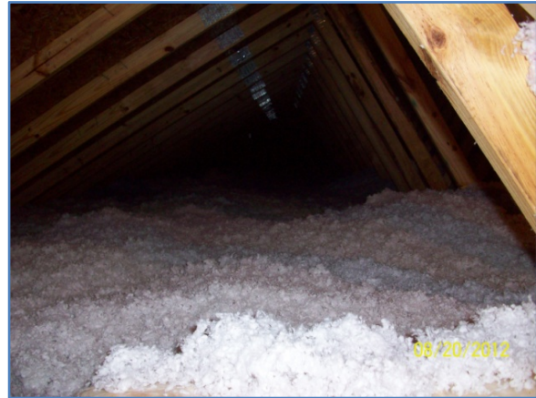
Figure 24. Buried ducts
