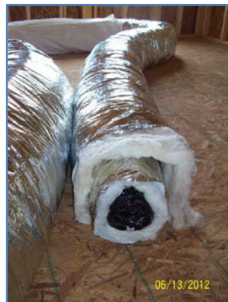
Figure 22. Flexible branch "duct within a duct"
