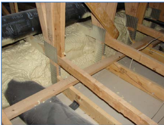
Figure 15. Encapsulated supply trunk
