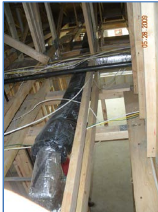
Figure 14. Supply duct layout
