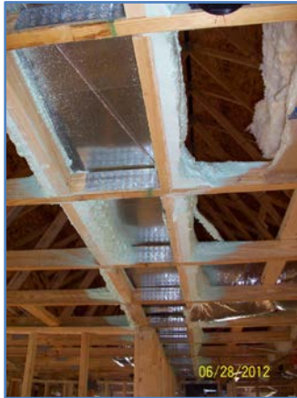
Figure 23. Encapsulated supply trunk before drywall
