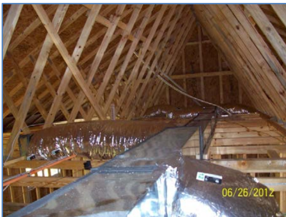
Figure 21. Second-floor supply trunk and compact duct layout
