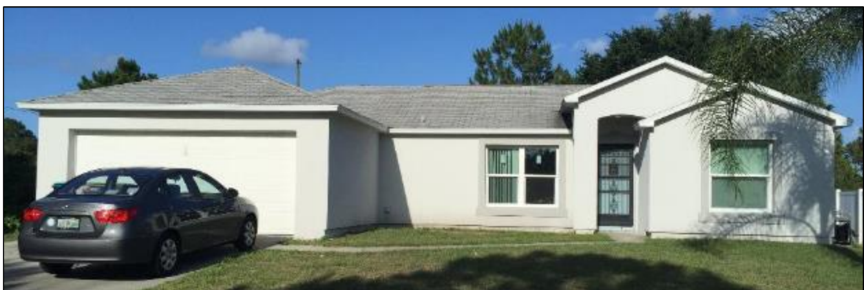
Figure 30. Site 54 after the exterior insulation finish system and window retrofit
