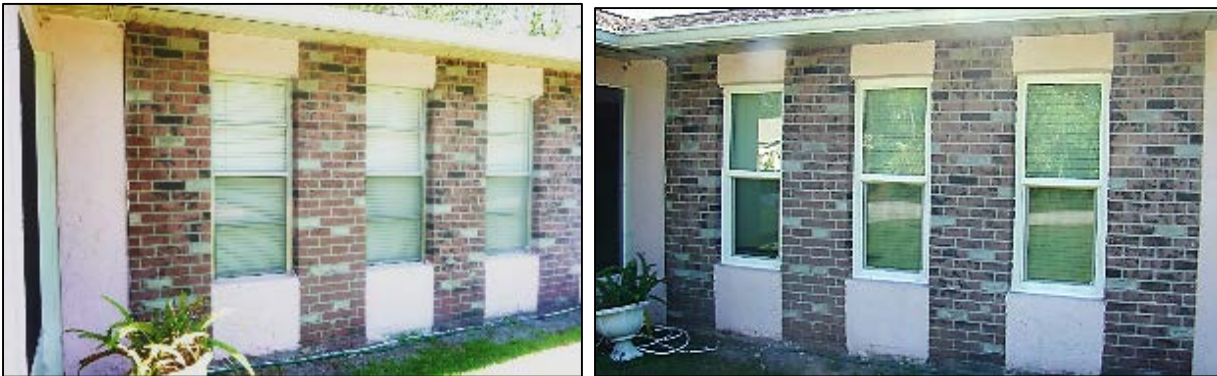
Figure 21. Site 23 window retrofit, pre-retrofit with existing single-pane, metal-framed windows (left), post-retrofit with double-pane, vinyl-frame windows (right)
