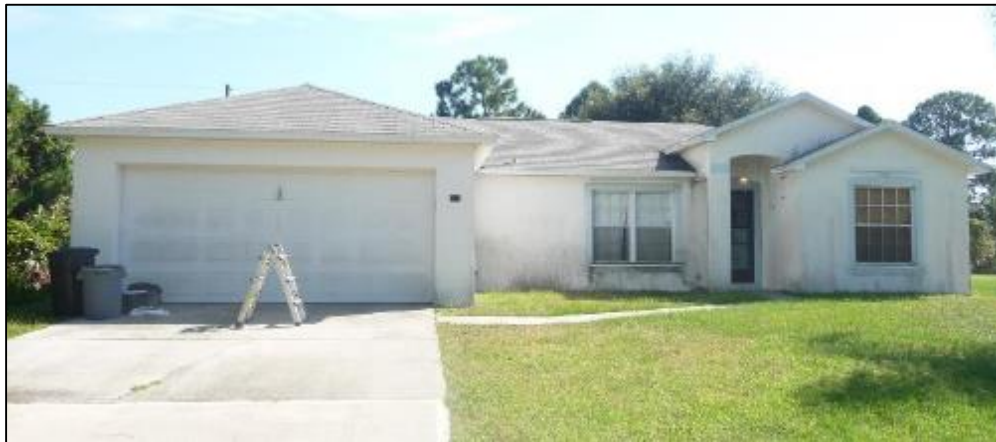
Figure 13. Site 54 Prior to EIFS and window retrofit
