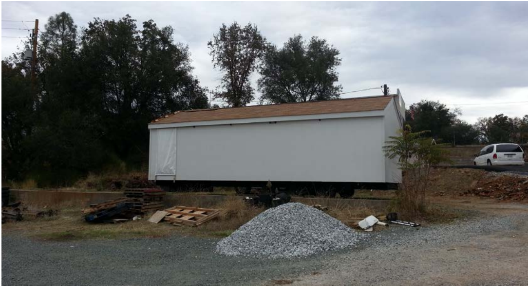
Figure 12. Test unit on-site—west façade
