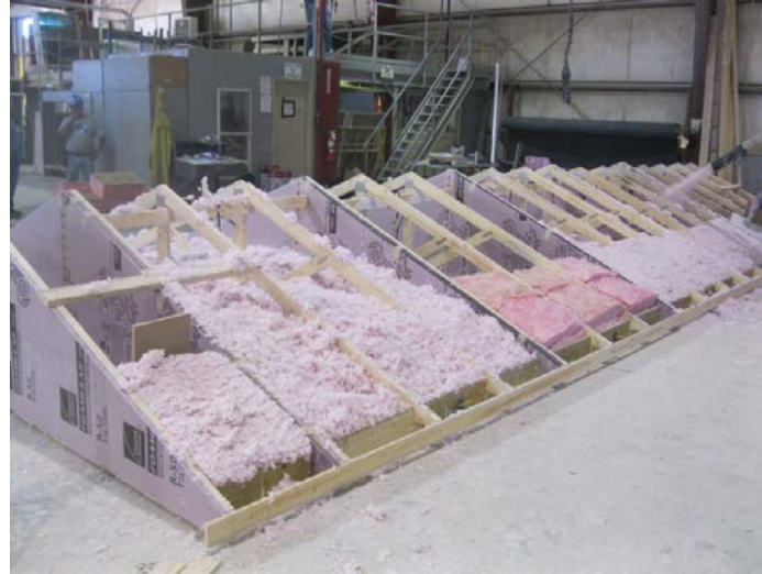
Figure 1. Roof test apparatus under construction
