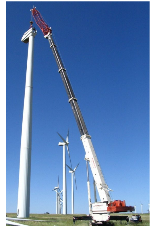
GRC field testing. Jeroen van Dam, NREL 19257
