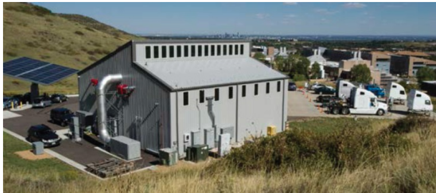
Figure 2. The Vehicle Testing and Integration Facility. Photo by Dennis Schroeder, NREL 31843
