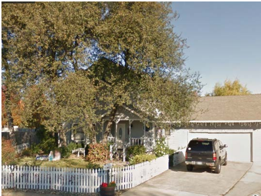
Figure 3. Street view of Site 2
