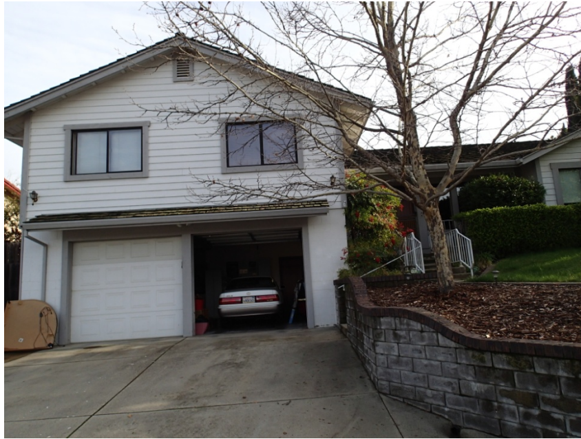
Figure 2. Street view of Site 1
