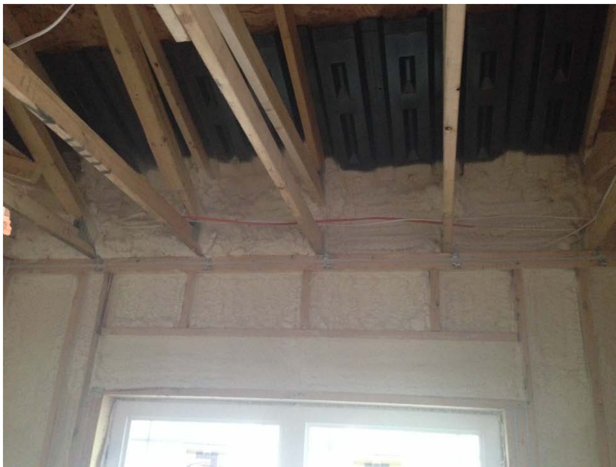
Figure 18. Amaris Custom Homes: Spray foam walls and energy heel truss of the White Bear Township, Minnesota, project
