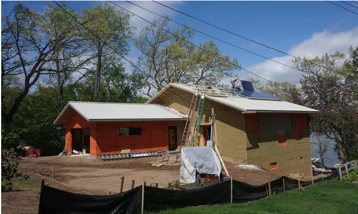
Figure 27. Morrissey Builders: Solar panel installation of the Lake Elmo, Minnesota, project
