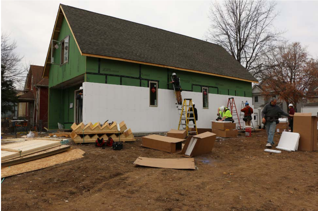
Figure 31. Urban Homeworks: Expanded polystyrene continuous insulation with embedded polypropylene attachment studs of the North Minneapolis, Minnesota, project
