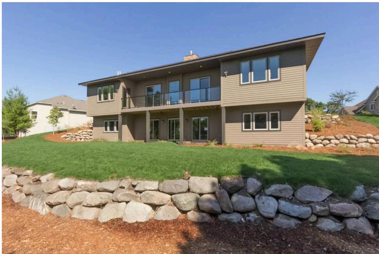
Figure 2. Amaris Custom Homes: Rear elevation of the St. Paul, Minnesota, project
