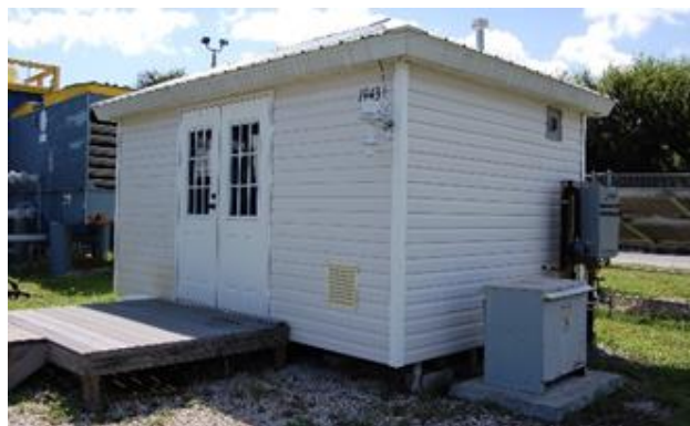
Figure 1. The HWS laboratory is a 160 ft 2 building with metal roof, housing seven systems and one externally-mounted tankless water heater.
