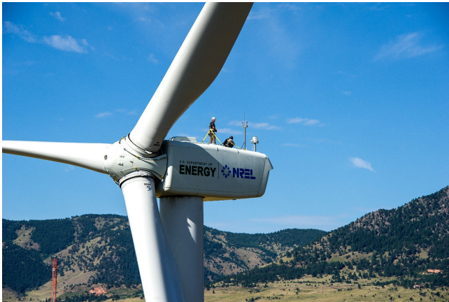
Figure 1. GE 1.5/77sle turbine at the National Wind Technology Center. Photo credit: Dennis Schroeder, NREL (image gallery number 29611).
