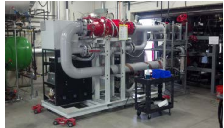
Access Energy XLT 125 kW Integrated Power Module
