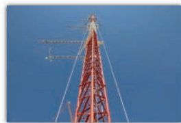
Monitoring using a 135-meter meteorological tower at the NWTC. Photo by Lee Jay Fingersh, NREL 40950
