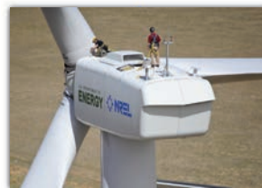
Testing on the U.S. Department of Energy 1.5-MW wind turbine at the NWTC. Photo by Lee Jay Fingersh, NREL 19007
