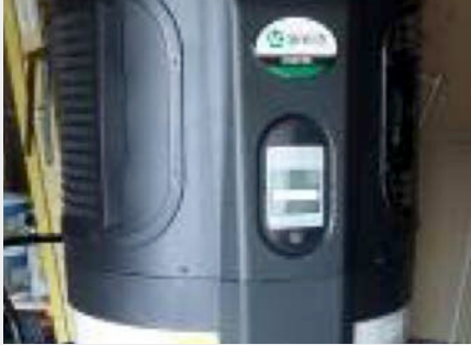
At nine sites, heat pump water heaters replaced electric resistance tanks.
