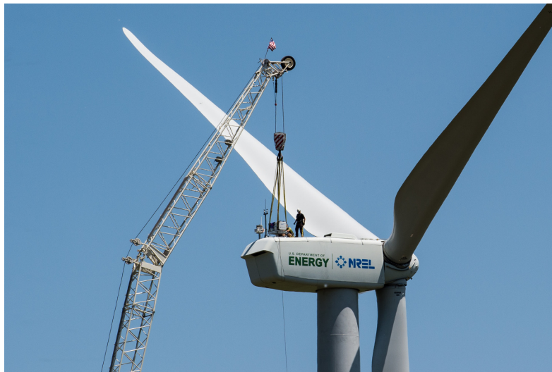
Figure 1: The U.S. Department of Energy (DOE) 1.5 turbine at the National Wind Technology Center is shown with the University of Stuttgart lidar being installed. Photo by Dennis Schroeder, NREL 38271
