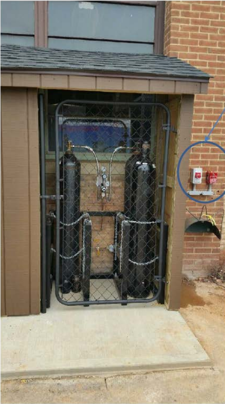
Figure 6. Location of fire alarm pull box. Figure from Proton OnSite
