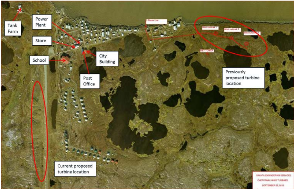
Figure 2-3: Aerial view of Chefnak. Source: Dennis Meiners
