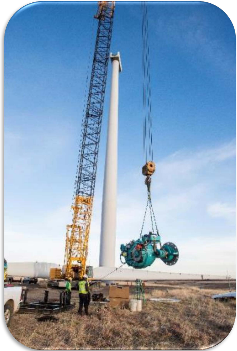
U.S. Department of Energy 1.5 rotor removal/gearbox swap at the National Wind Technology Center. Photo by Dennis Schroeder, NREL 49407
