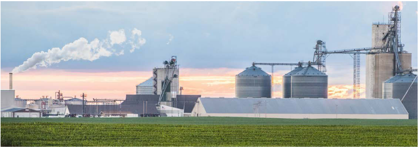
Plants like this one in Nevada, Iowa, commonly use dry mill technology to process corn into fuel-grade ethanol and distiller's grains. Photo by Dennis Schroeder, NREL 47103
