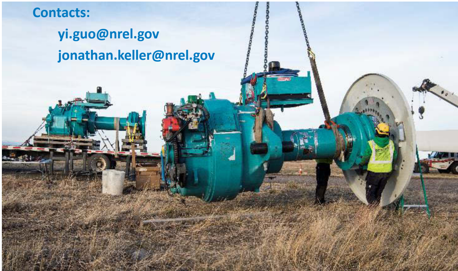
Photo by Dennis Schroeder, NREL 49418
