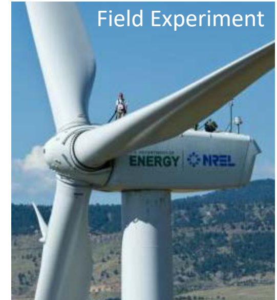
Photo by Dennis Schroeder, NREL 21864
