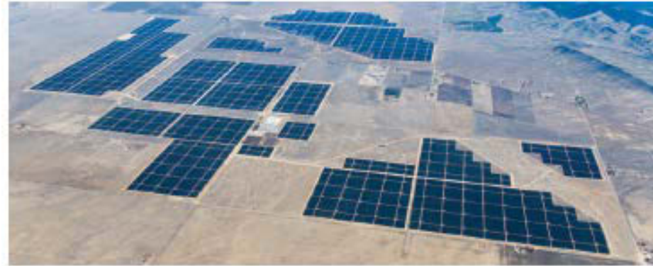
550 MW PV Plant [4]
