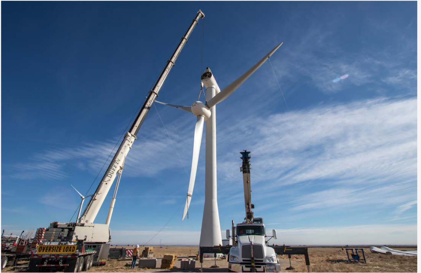
Higher hub heights make it possible to cost-effectively tap wind resources beyond the reach of today's typical turbines. Photo by Lee Jay Fingersh, NREL 54225
