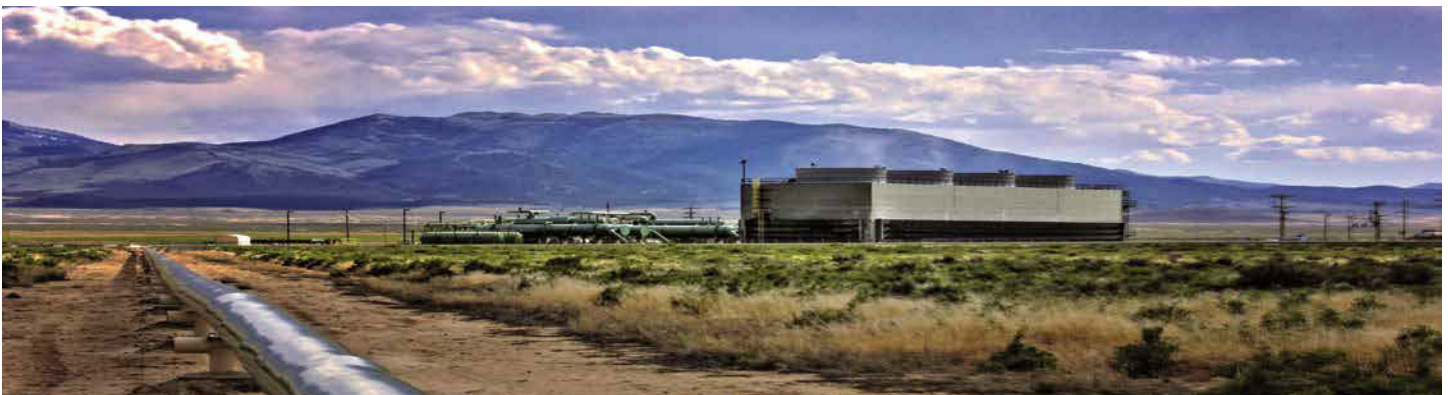
Raft River geothermal power plant in Idaho. Photo credit: Roxie Crouch
