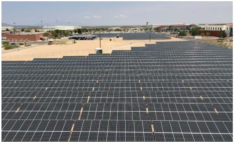
DEA's 2.5 MW-DC PV system helps the agency meet energy-related mandates for federal facilities and saves approximately $288,000 annually (nominal dollars).
