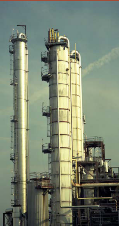
Photo by Warren Gretz, NREL 282
