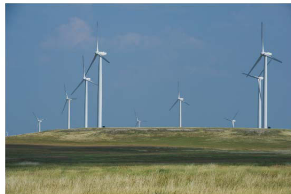
Photo by Dennis Schroeder, NREL
