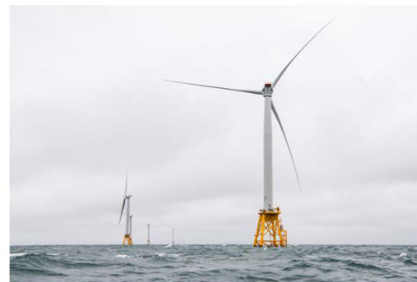
Photo by Dennis Schroeder, NREL
