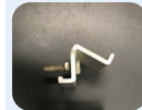
Photo showing bent end clamp recovered from a PV site after a hurricane. Photo from Andy Walker, NREL
