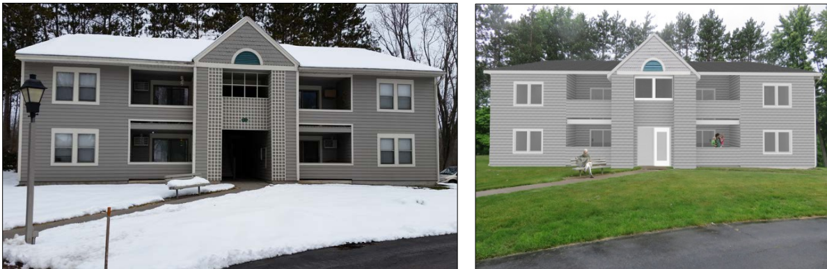
Figure 4 – Christopher Court existing building (L) and rendering of post-retrofit (R). The rendering is a simplified version of the building; there are no plans to remove windows. Photo courtesy: Rock PMC; Rendering courtesy: King + King Architects
