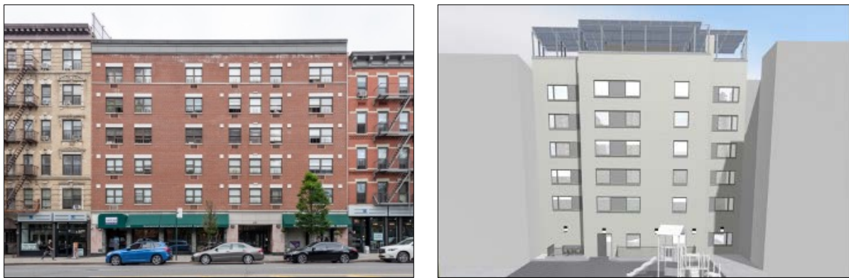
Figure 2 – The Levy Partnership existing building (L) and rendering of post-retrofit (R) Photo courtesy: “RetrofitNY: The Levy Partnership Net Zero Energy Schematic Design” (NYSERDA 2019) Rendering courtesy: CTA Architects P.C.
