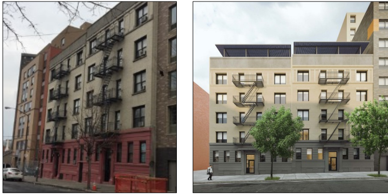
Figure 3 – Bright Power existing building (L) and rendering of post-retrofit (R) Photo courtesy: “RetrofitNY: Bright Power Net Zero Energy Retrofit Schematic Design” (NYSERDA 2019) Rendering courtesy: Magnusson Architecture & Planning P.C.
