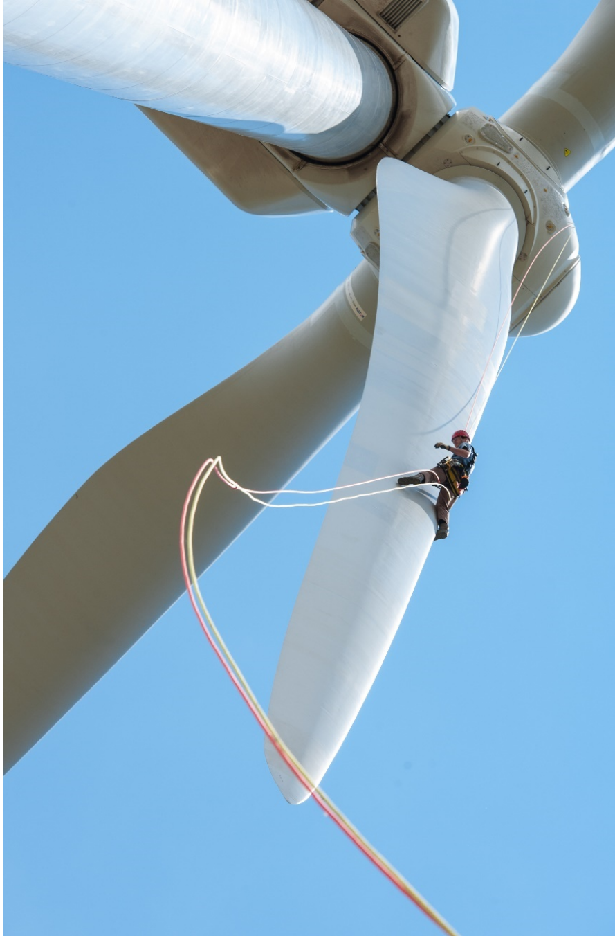
Figure 17. Rope workers installing tufts on the Alstom ECO110 blades (NREL PIX: 27196)
