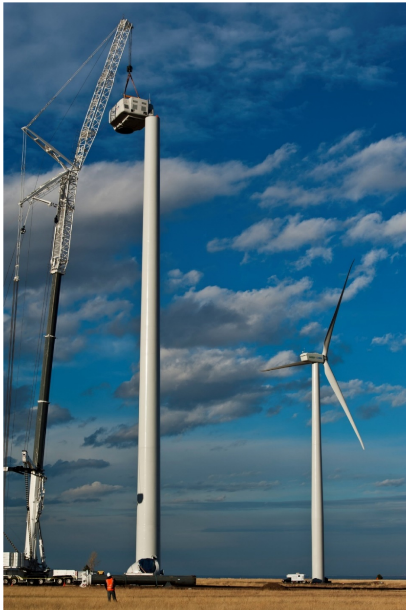
Figure 1. Installation of the ECO100 nacelle
