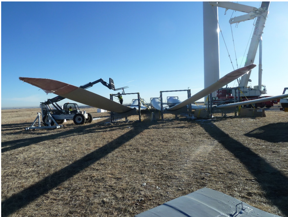
Figure 11. AL 53 blades being prepared for installation on the ECO100 wind turbine
