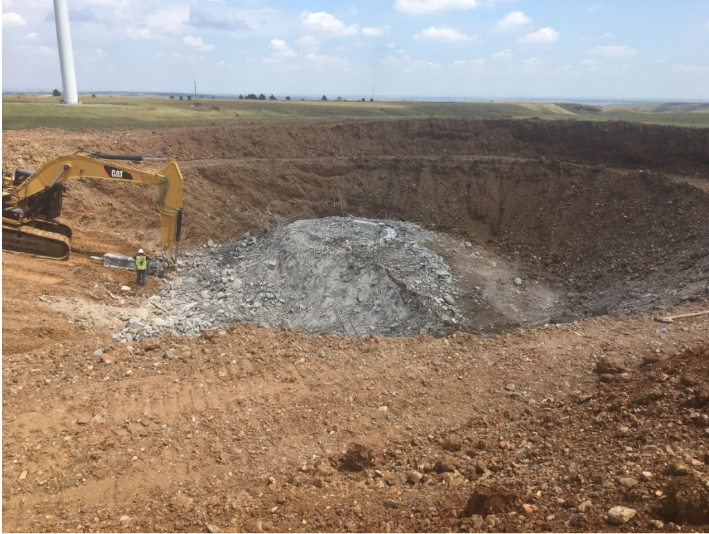
Figure 6. Foundation removal
