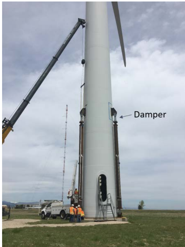
Figure 21. Installation of tower dampers
