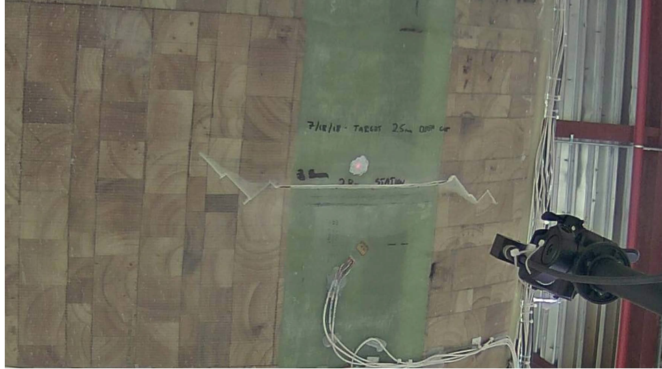
Figure 2. Blade damage on low-pressure spar cap at the 2.8 m station
