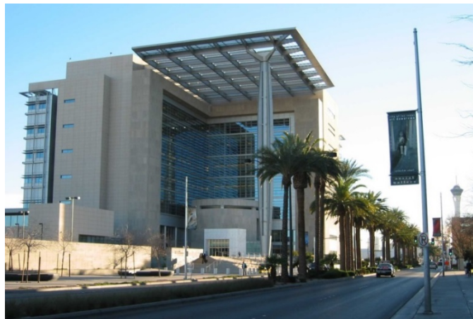
Figure 12. Picture of the Lloyd D. George Federal Building (Credit: Gregg Tomberlin, NREL)
