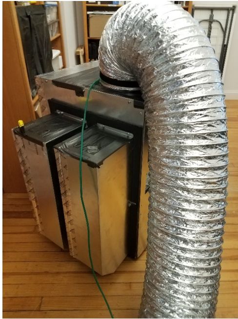
Figure 29. The entire cabinet was sealed and leak tested using a Duct Blaster
