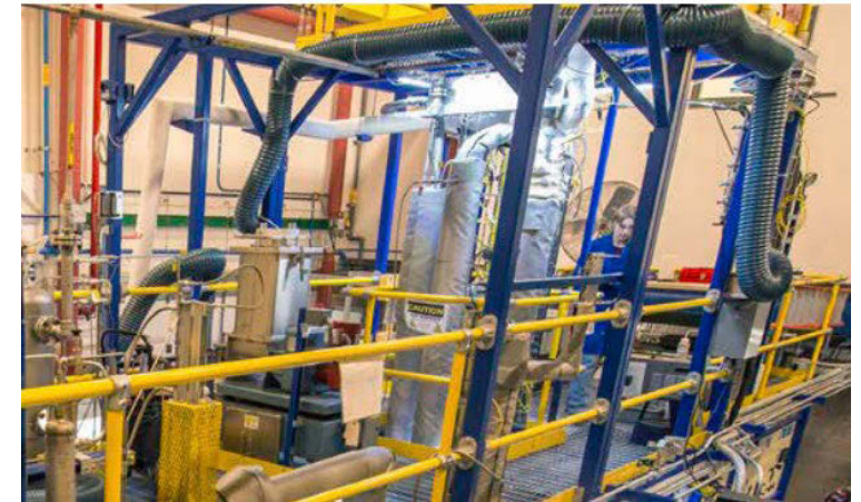
Davison Circulating Riser* at NREL
