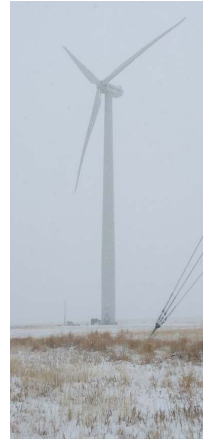
NREL GE 1.5 MW. Photo by NREL
