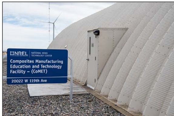
By Dennis Schroeder, NREL 41790
